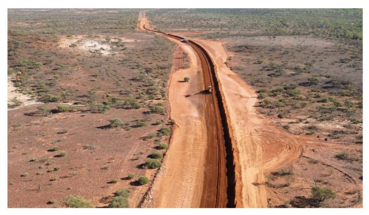
Figure 2: Basecourse being laid at end of existing seal.
