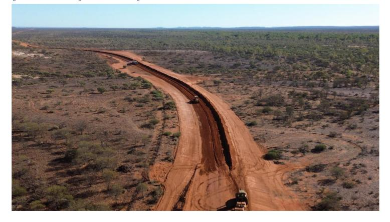
Figure 1: New basecourse through design section bends
