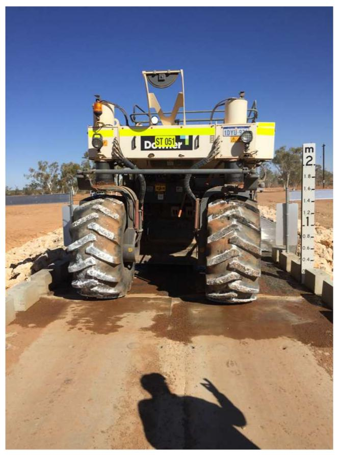
Stabilising Machine on Killili Bridge going to stabilise the approach on the south side of the bridge for more bitumen to be laid out on a small section of the road.
