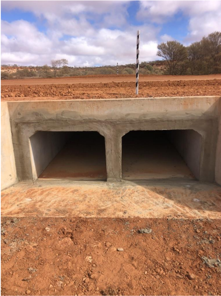
Figure 2: Culvert/ Headwall mortar in place
