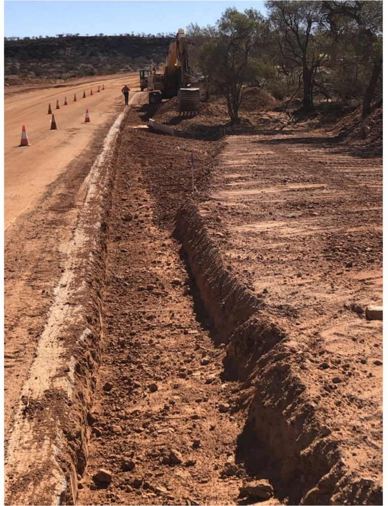
Figure 1: Box out for floodway rock protection.
