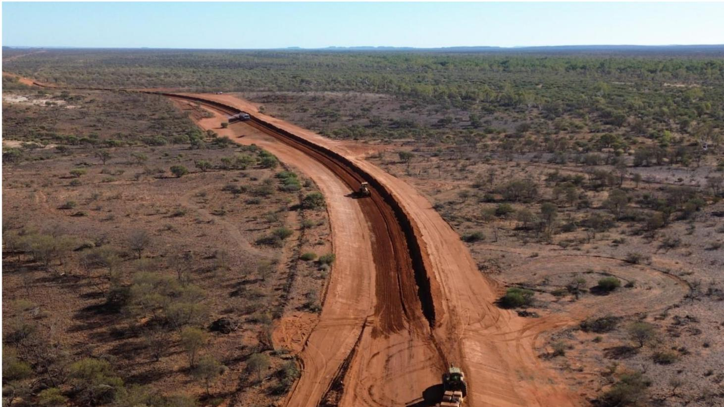
*Figure 1: New basecourse through design section bends*
