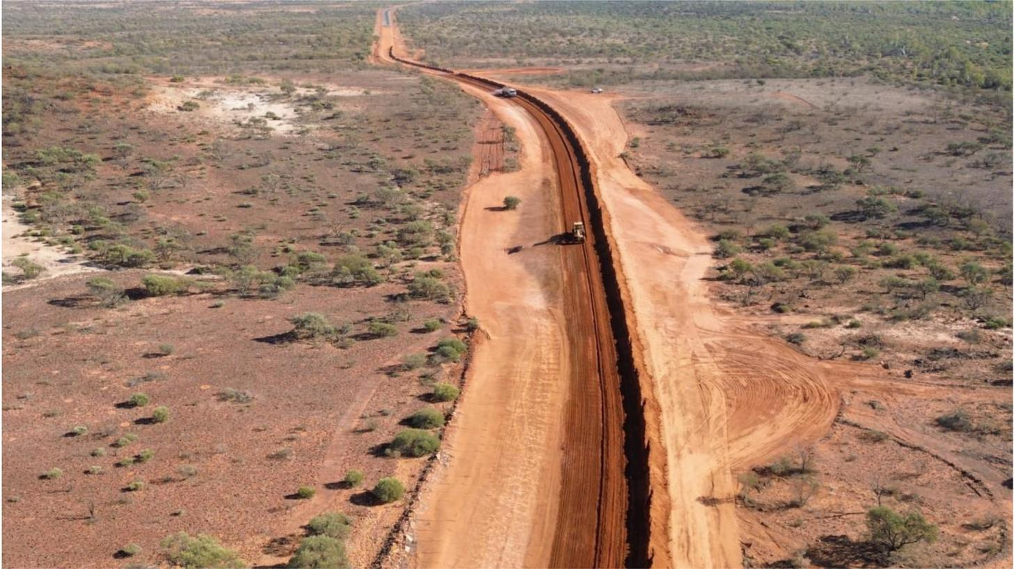
*Figure 2: Basecourse being laid at end of existing seal.*
