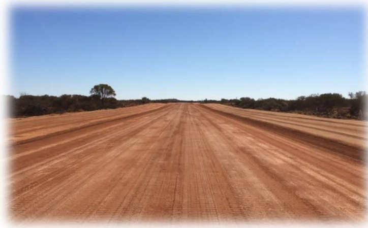
(Re-sheeting Ullawarra Road)
