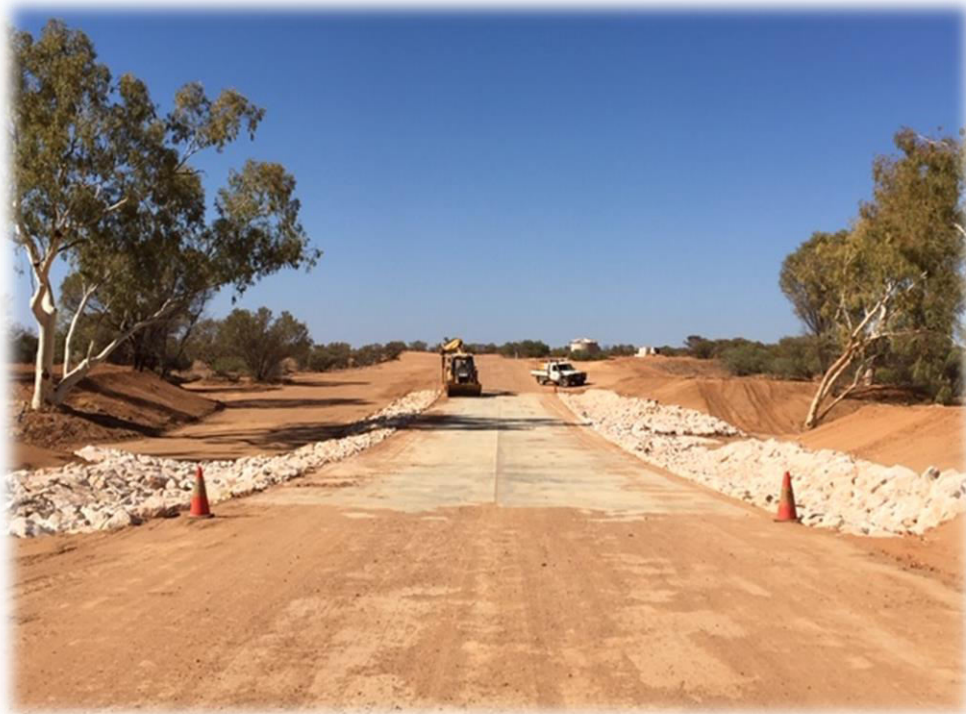
New Coordewandy crossing
