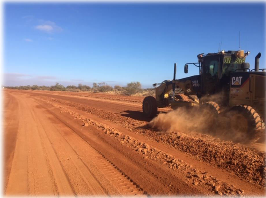
Shire reconstruction works on Ullawarra road
