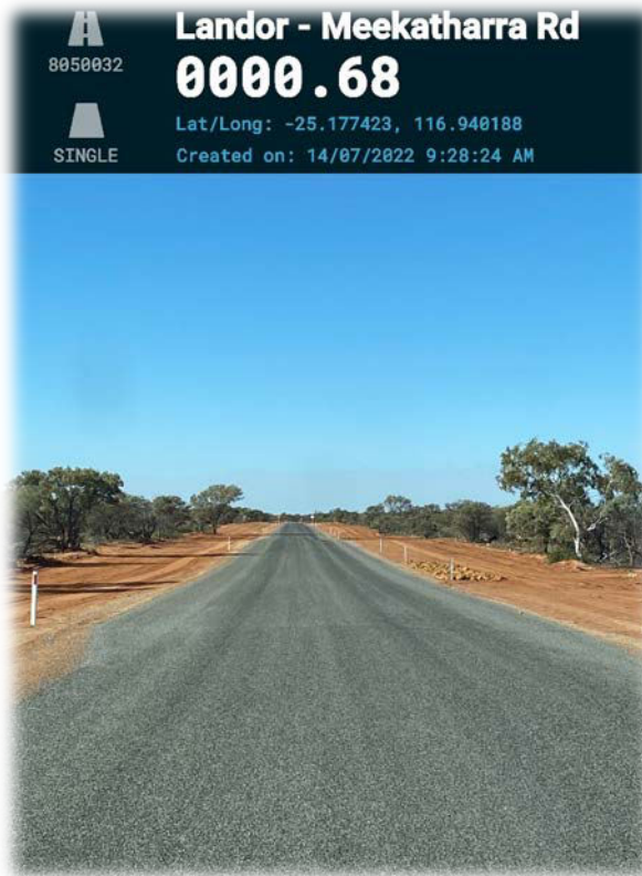
New bitumen seal and rock protection on Landor Meekatharra Road
