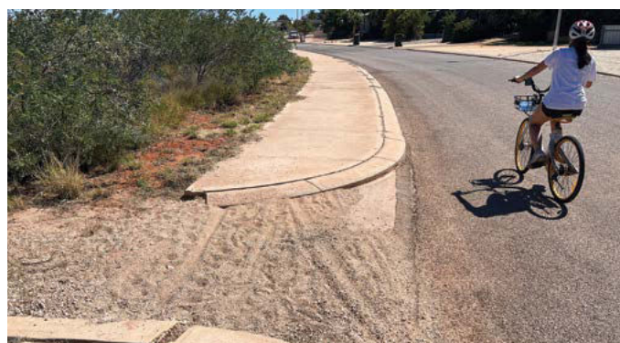
Drainage/spillway channels disrupting path continuity in Exmouth.
