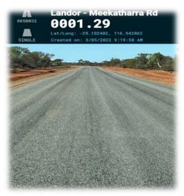
We have completed re-sheeting a two kilometre section of road in front of the Landor race course on Landor Mt Augustus road. Due to the condition of the road between the Landor homestead and race course we decided to water, roll and reshape this section as it was unsafe and to prevent further damage to the road. We will sheet a further 1.5km of rough road section on the south side of the Burringurrah Community once we have completed the backslopes on Landor Meekatharra road.
