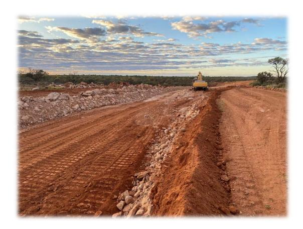
The works crew have all but completed the new bitumen seal on Landor Meekatharra road. We have some backslopes to finish this week. Due to issues with watercart availability, rain delays and an unnegotiable timeslot for the seal crew were only able to achieve 4.2km of new seal. However we have been able to prepare a further 3km of subgrade in preparation for our next campaign.
