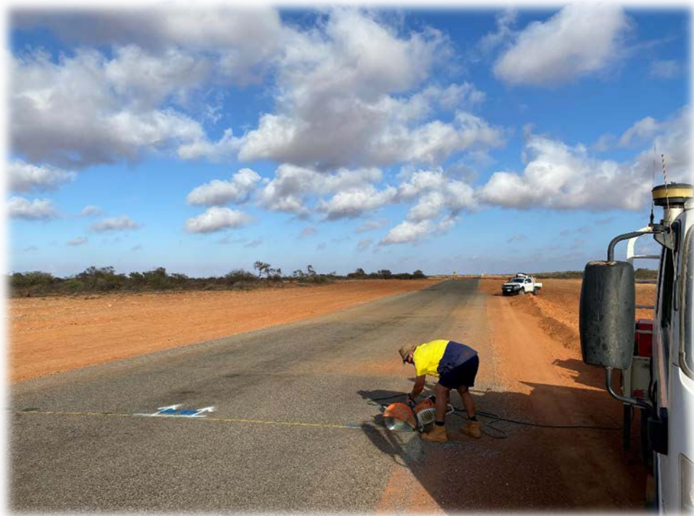
Figure 1 Preparing for restabilising and reforming floodway
