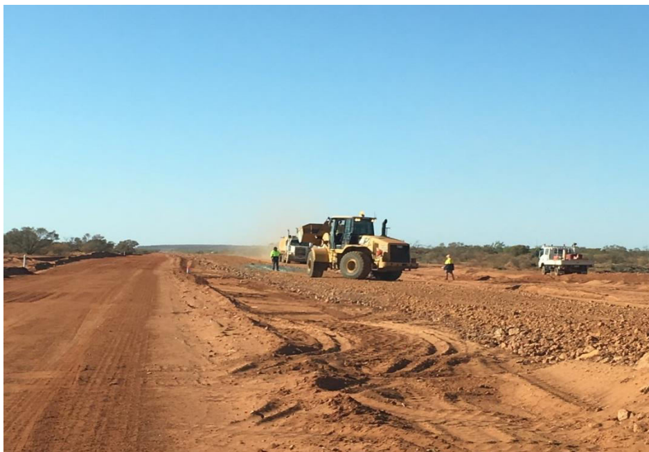
Figure 1: preparing for cement stabilisation of flood ways
