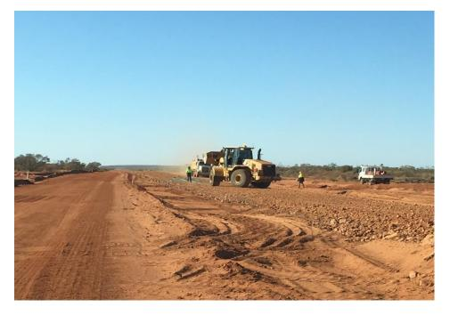
Figure 1: preparing for cement stabilisation of flood ways
