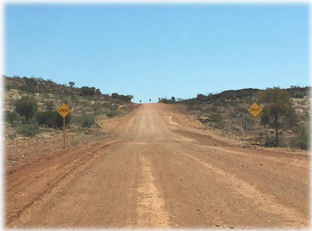
Figure 2: Cobra hill facing south.
