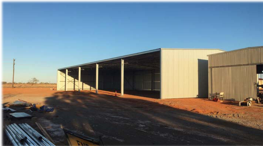
Figure 1: new machinery shed
