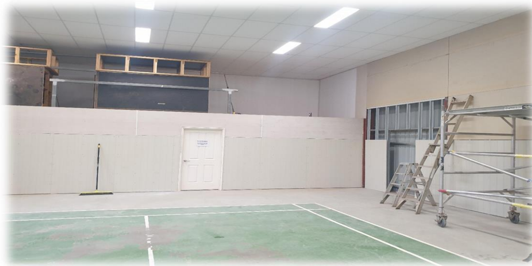
Figure 2: Newly cladded walls in the pavilion
