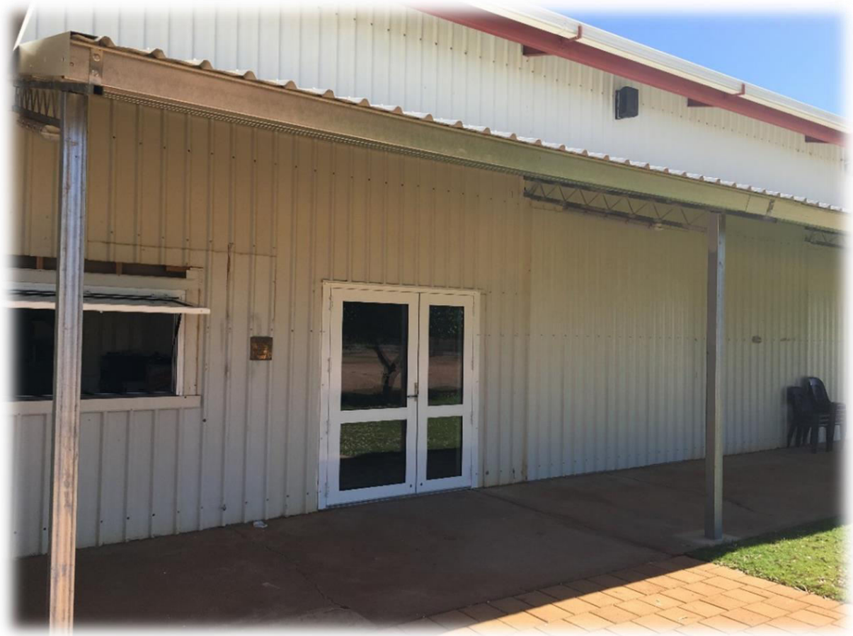
Figure 1&2: pavilion upgrades- new verandas and internal cladding.
