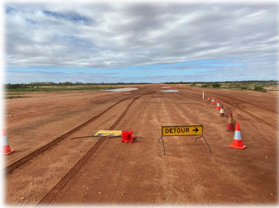
Figure 4 Road Closed sign run over and detour ignored on works prepared for bitumen
