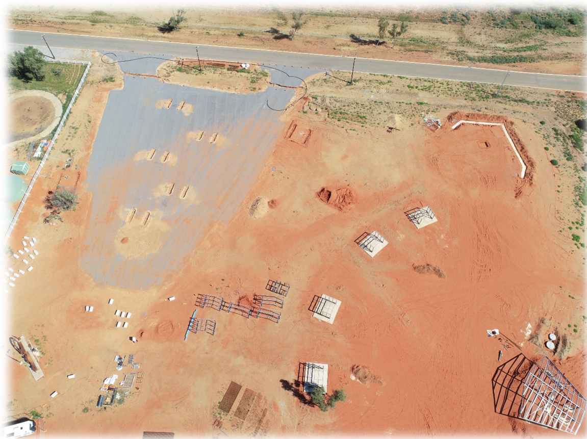
Figure 1: Visitor's Stop under construction.
