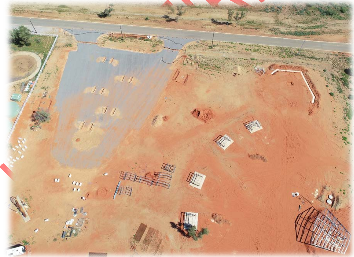
Figure 1: Visitor's Stop under construction.
