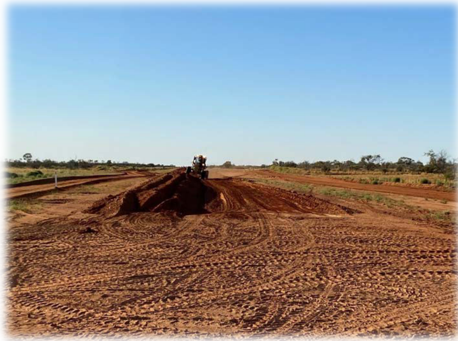
Figure 1 reconstructing the existing sub grade
