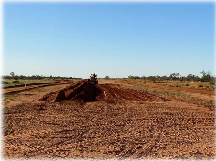
Figure 1 reconstructing the existing sub grade
