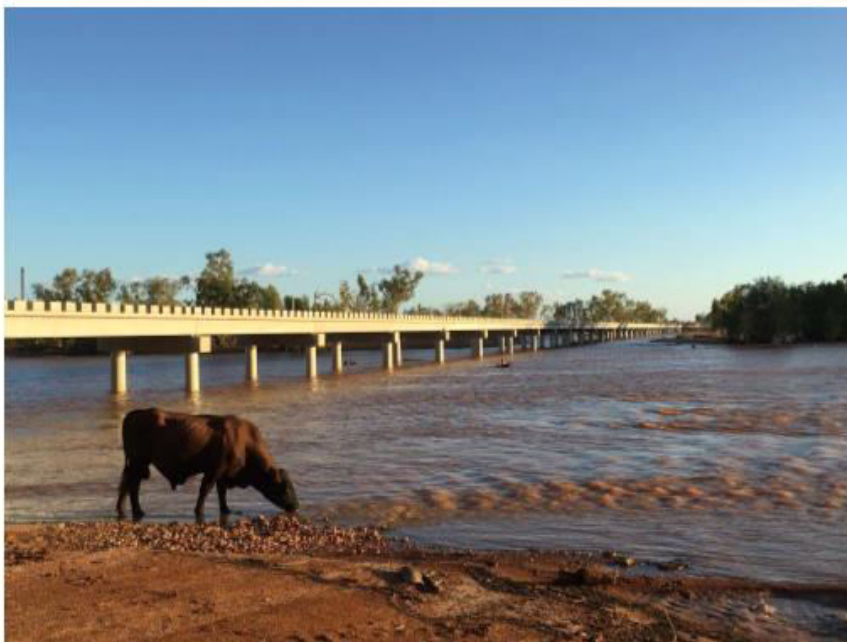
Killilli Bridge Opened December 2016 Photo Blanche Walker
