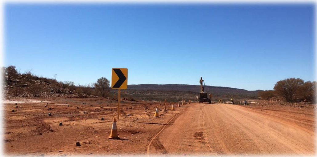
Figure 1-2: Drill rig on the Cobra hill.
