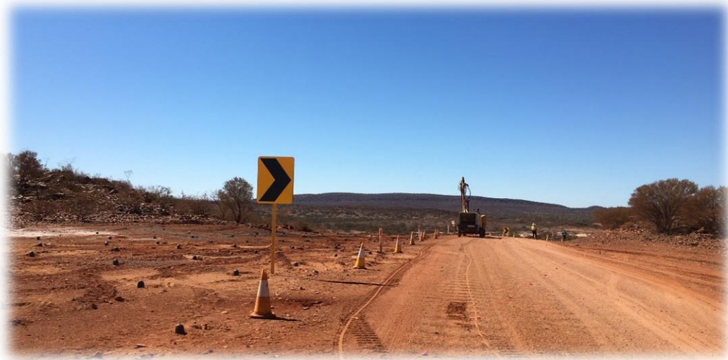
Figure 1-2: Drill rig on the Cobra hill.
