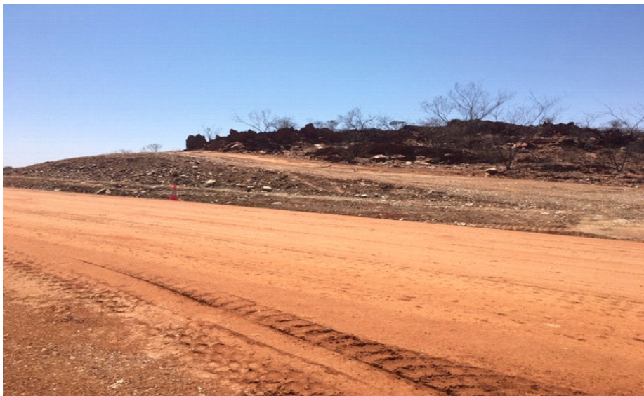
Figure 3 Burringurrah Hill- lowered 2m
