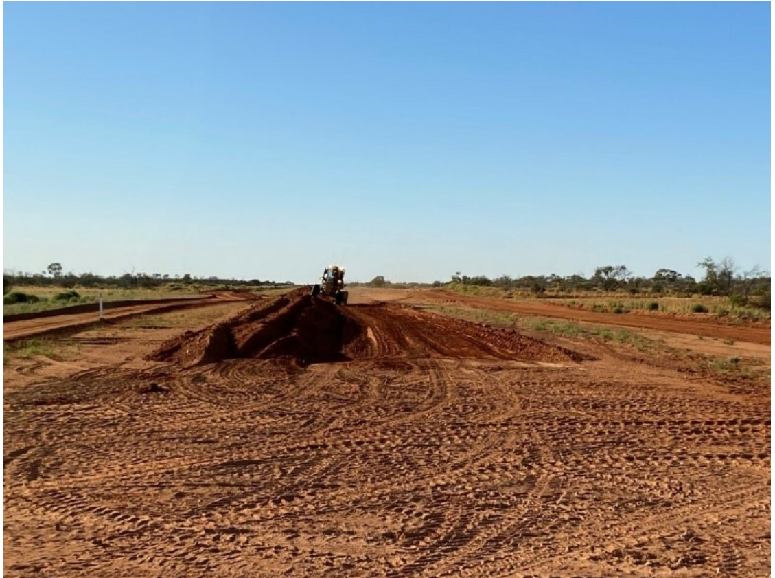
Figure 1: Reconstructing the Existing Sub Grade
