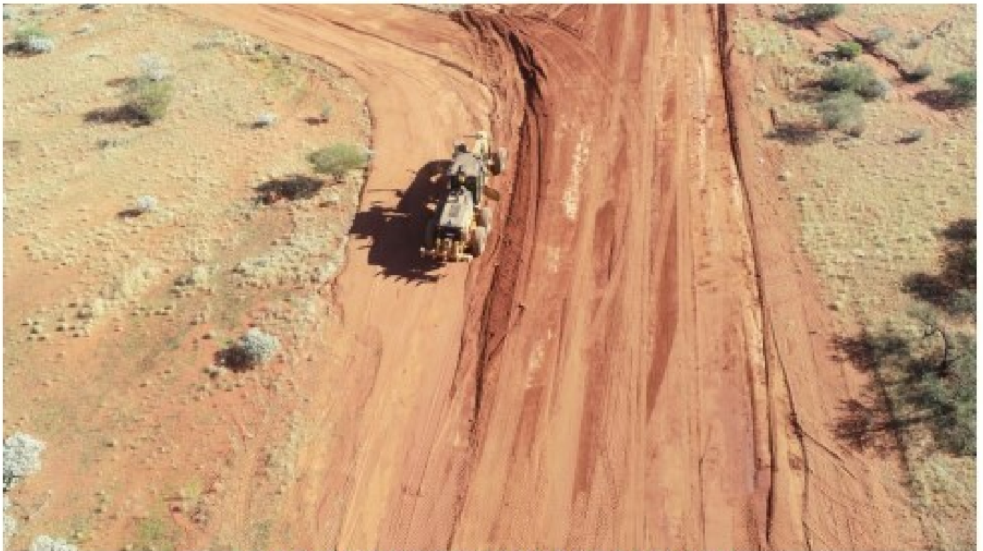
Landor Mt Clere Rd – Flood damage repair works
