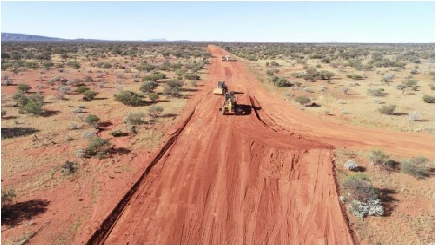
Grading works on Landor Mt Clere Rd
