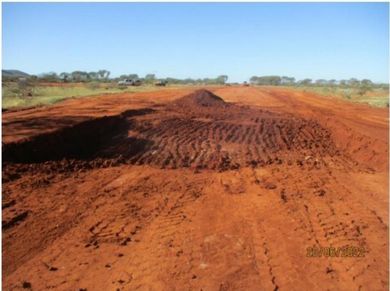
Gravel Resheet Rd – Defect repair works
