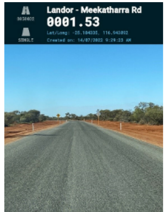
New bitumen seal and rock protection on Landor Meekatharra Road
