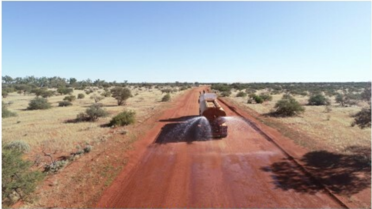
Landor Mt Clere Rd - Defect rectification works
