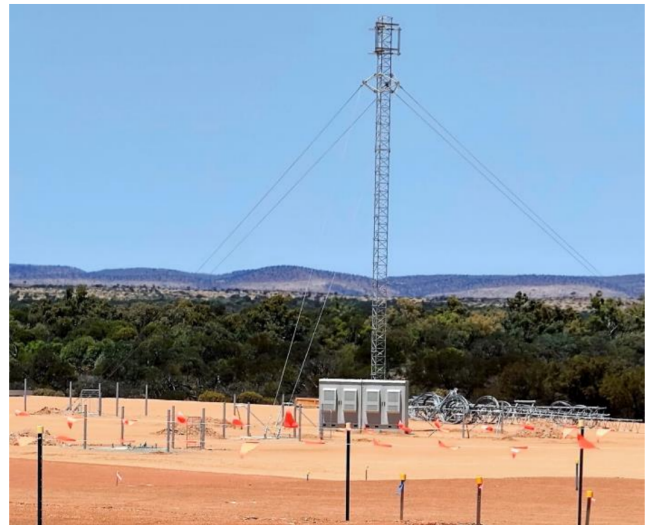
High speed network access to be delivered to site using point to point, line of sight microwave technology utilising existing and Hastings built towers spanning a 300 kms..
