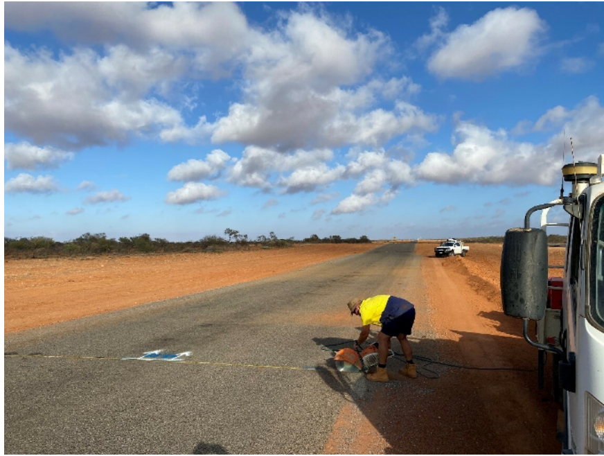
Figure1 Preparing for restabilising and reforming floodway
