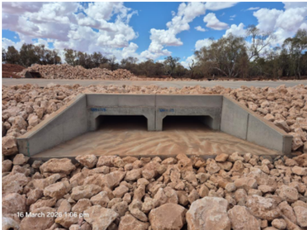
Work Area 5: Gascoyne River Floodway - Downstream Culvert and Rock Protection
