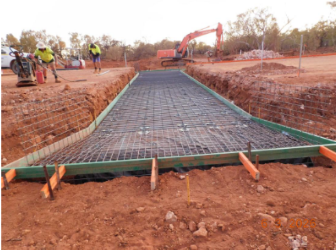
Work Area 5: Gascoyne River Floodway - Downstream Culvert Progress
