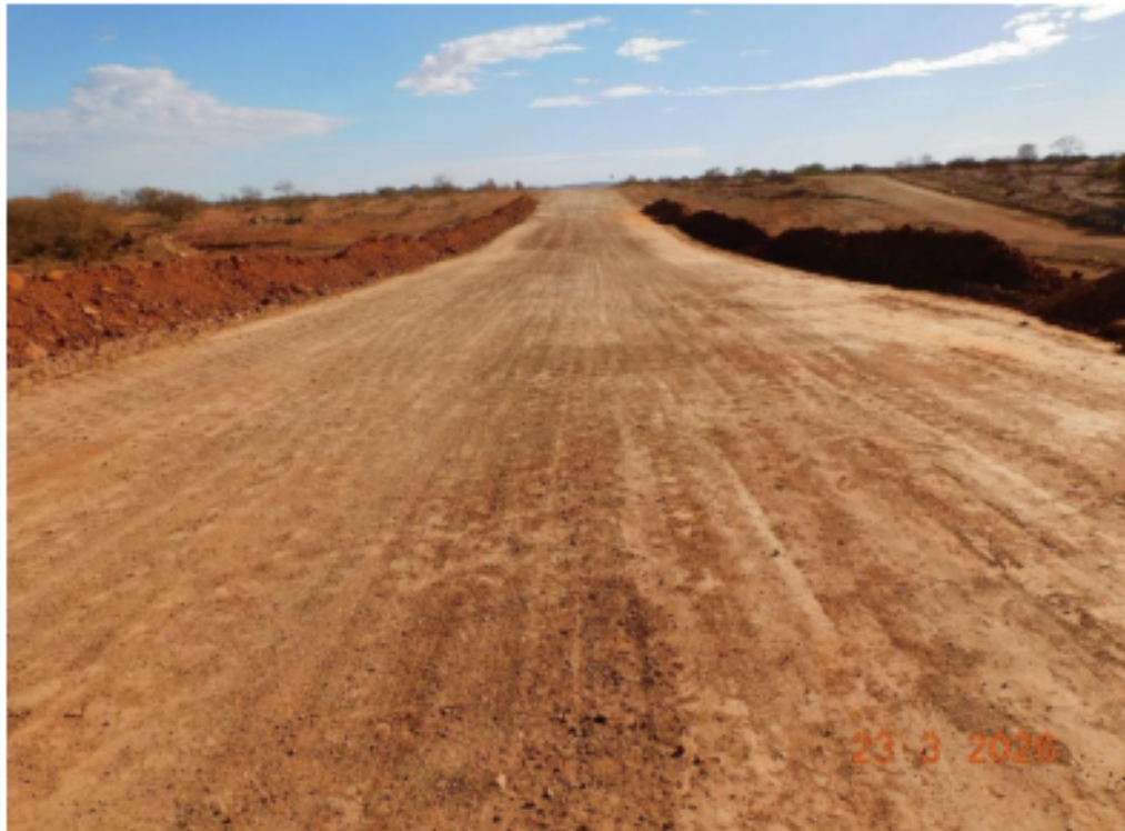
Work Area 8 (Pink Hills 2 nd Culvert Structure): Embankment Lift 3
