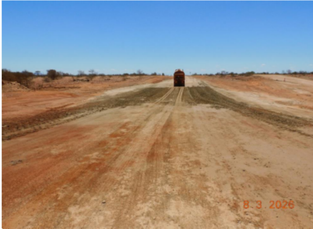
Work Area 8 (Pink Hills 2 nd Culvert Structure): Embankment Lift 2
