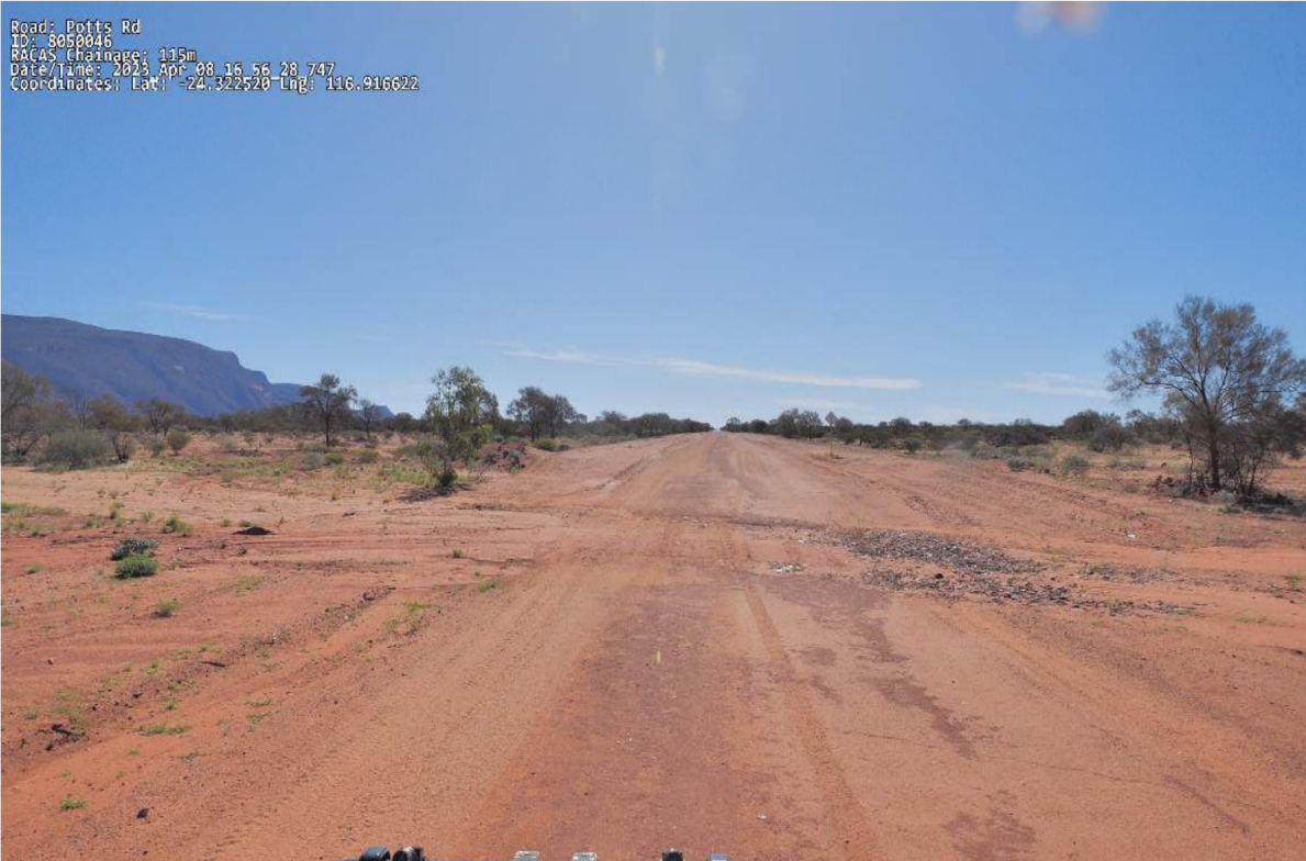
Potts Rd Slk 0.115-0.133 - Defect
