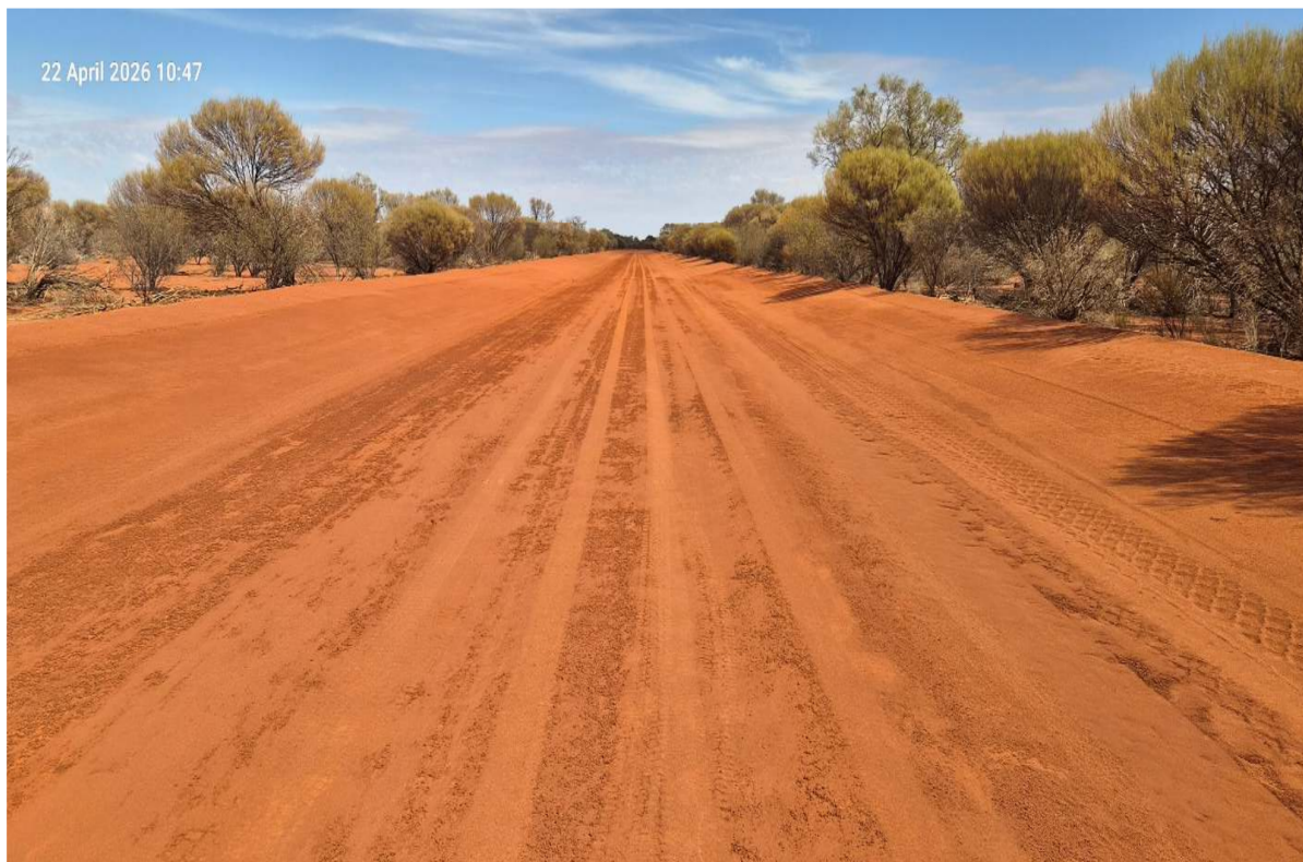
Mt Augustus Rd Slk 2.353-2.393 – Repair
