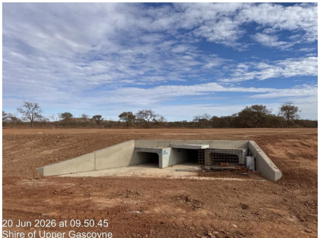
Pink Hills Culvert (Slk 64.5) culvert structure complete
