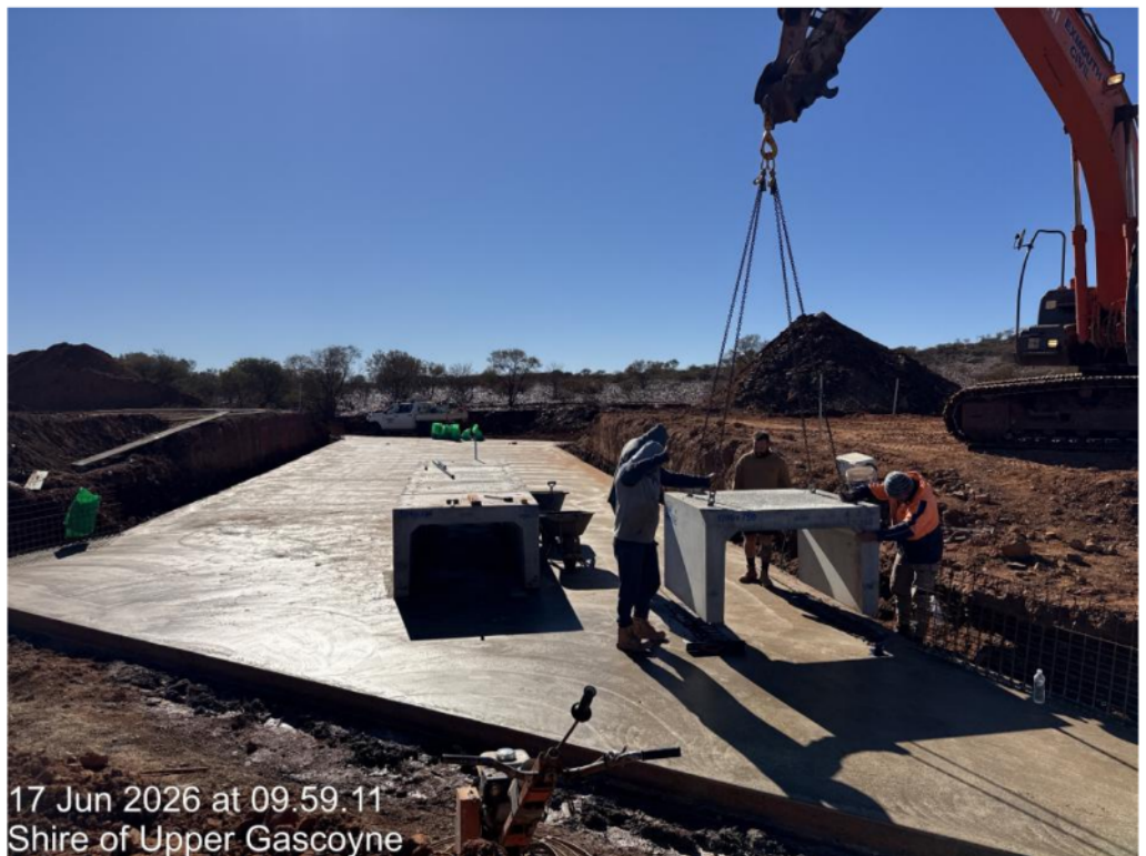
Pink Hills Culvert (Slk 78) base slab and first crown units
