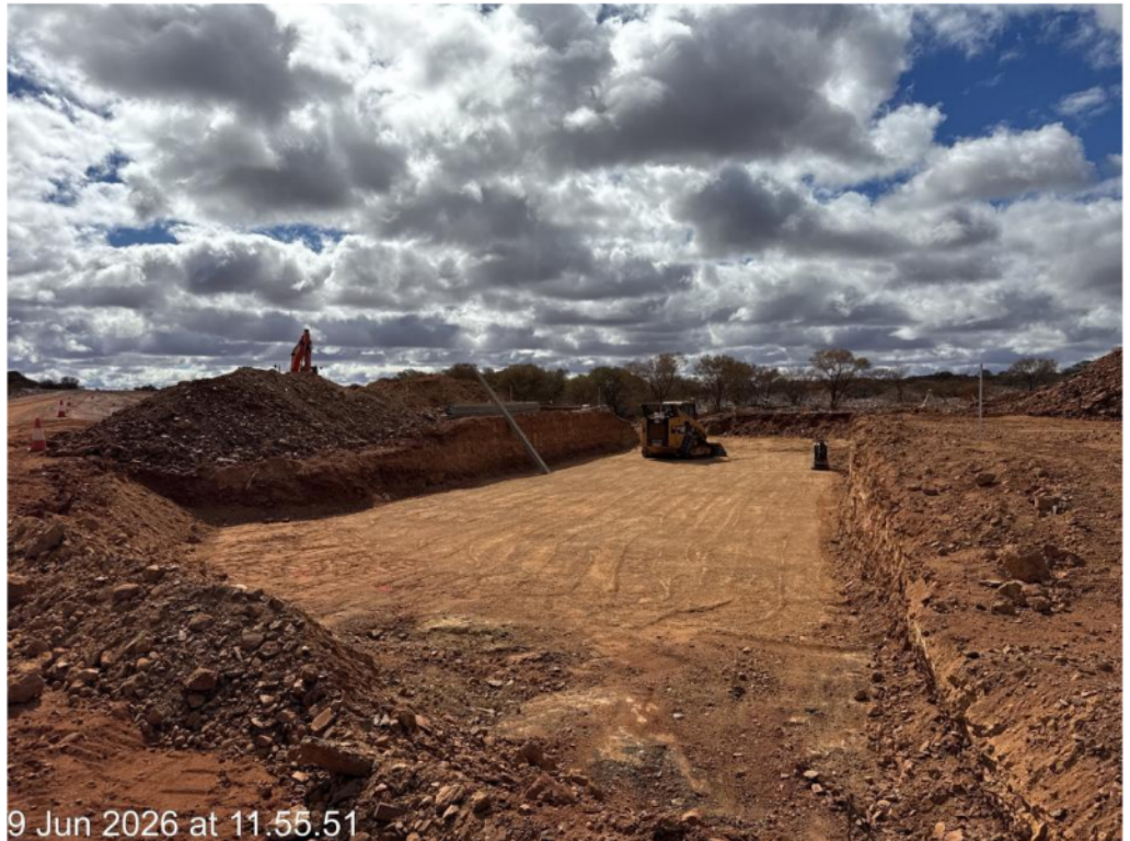
Pink Hills Culvert (Slk 78) excavation for base slab
