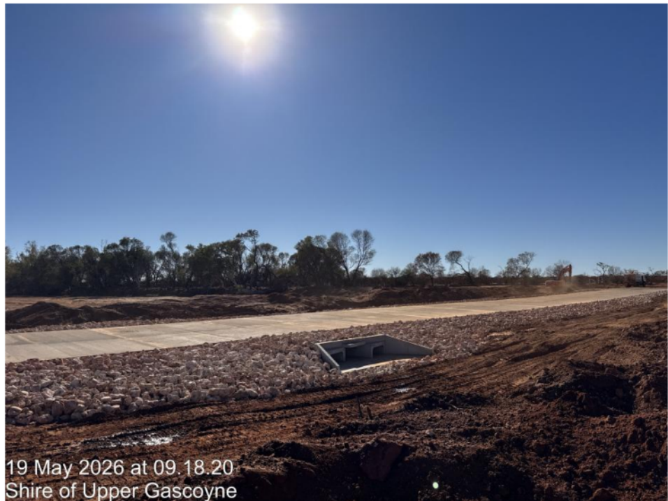
Aurilla Creek concrete floodway, culverts and scour protection complete
