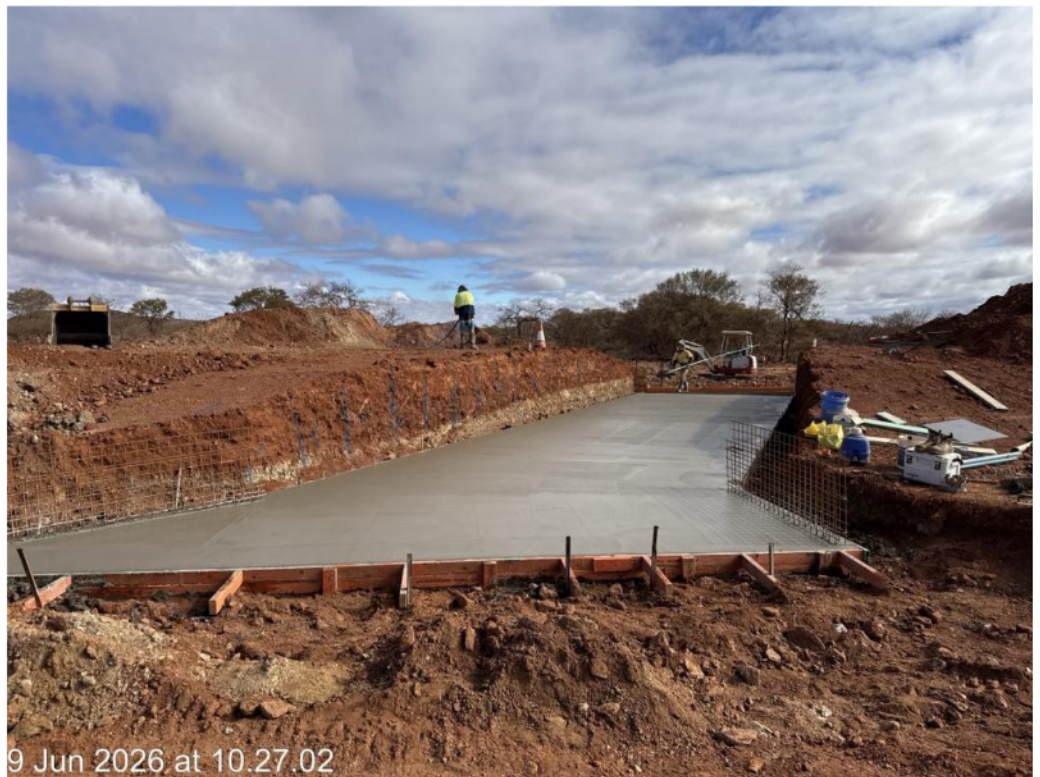
Pink Hills Culvert (Slk 64.3) base slab
