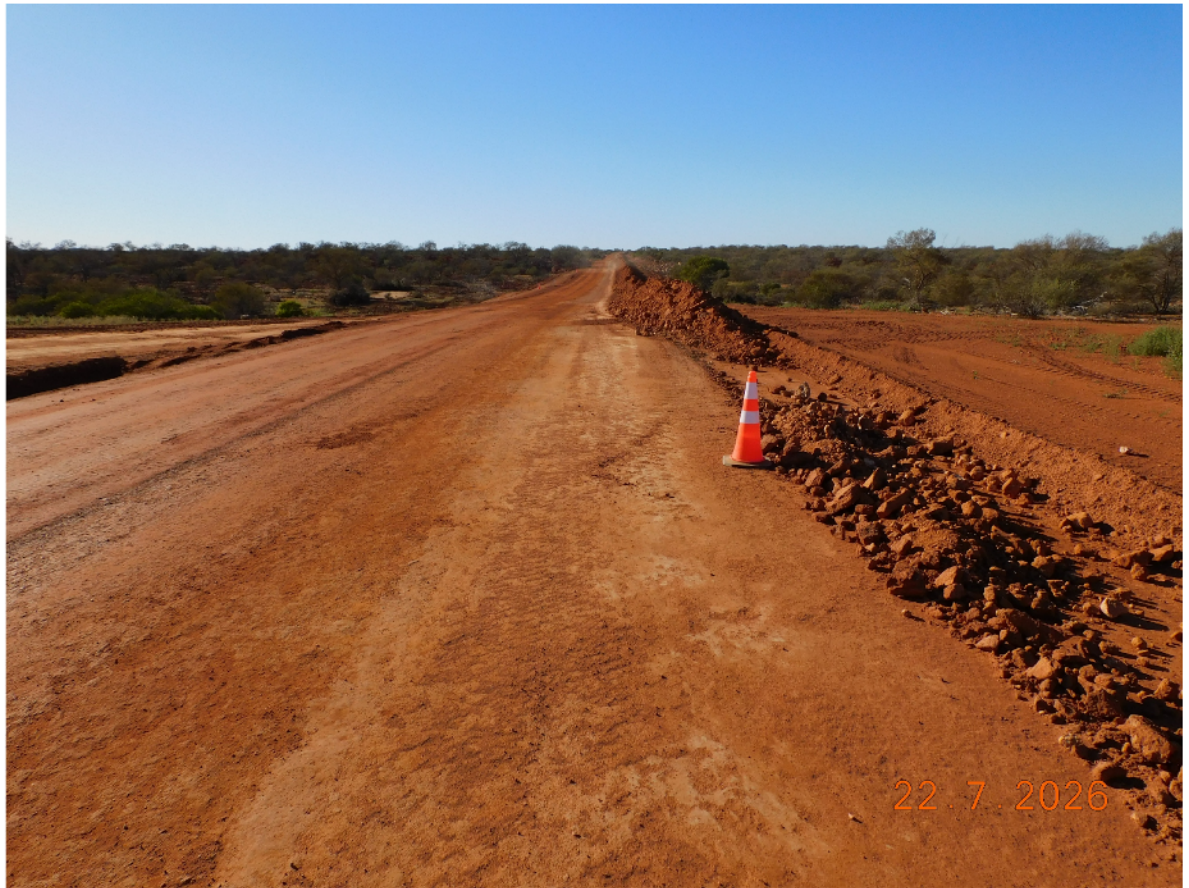
Tipping Out Basecourse
