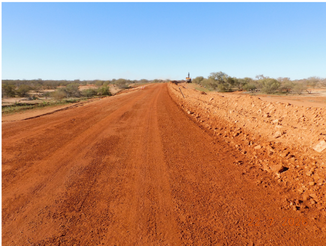
Tipping Out Basecourse
