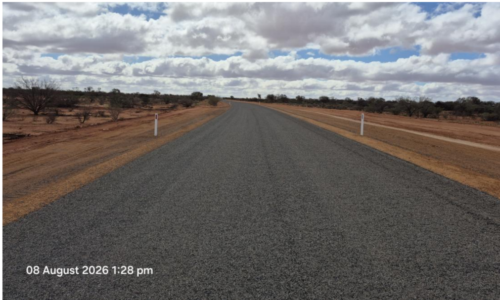
Work Area 2 - Landor Mt Augustus Rd realigned section south of Landor Mt Clere Rd
