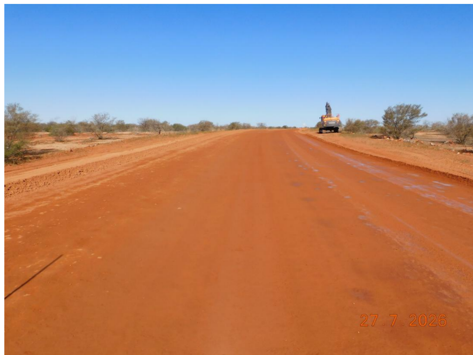
Basecourse ready for final trim and face up
