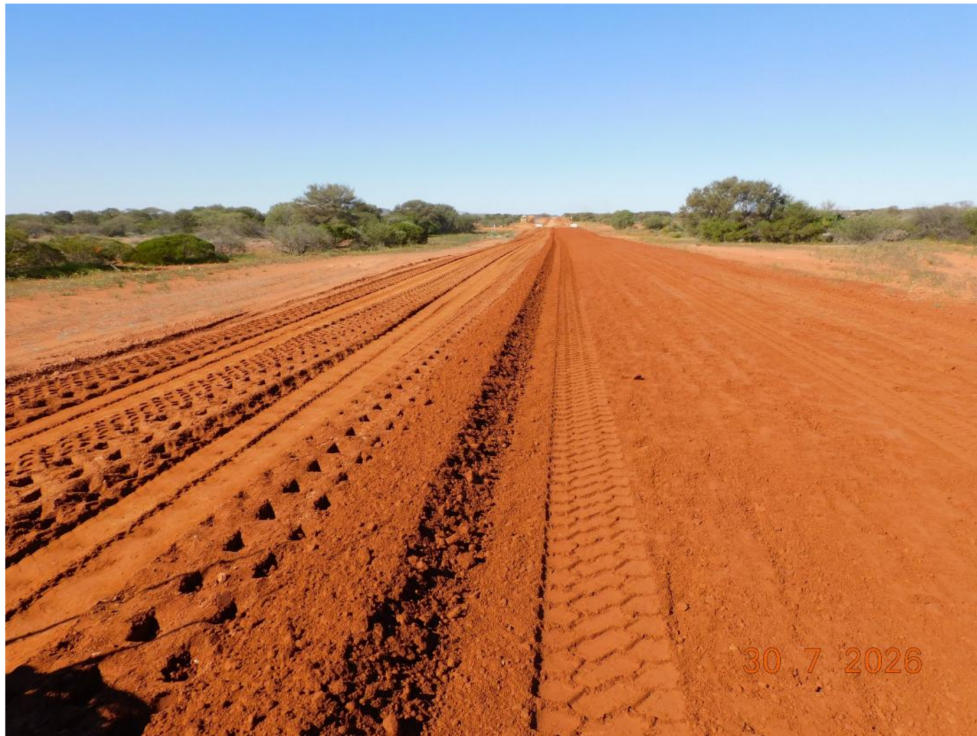
Basecourse mixing in progress
