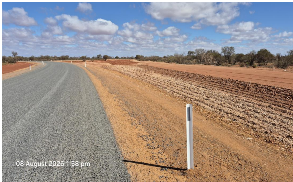
Work Area 1 - Landor Mt Augustus Rd north of Homestead ripped for rehabilitation
