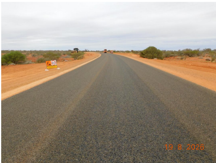
Completed two coat seal
