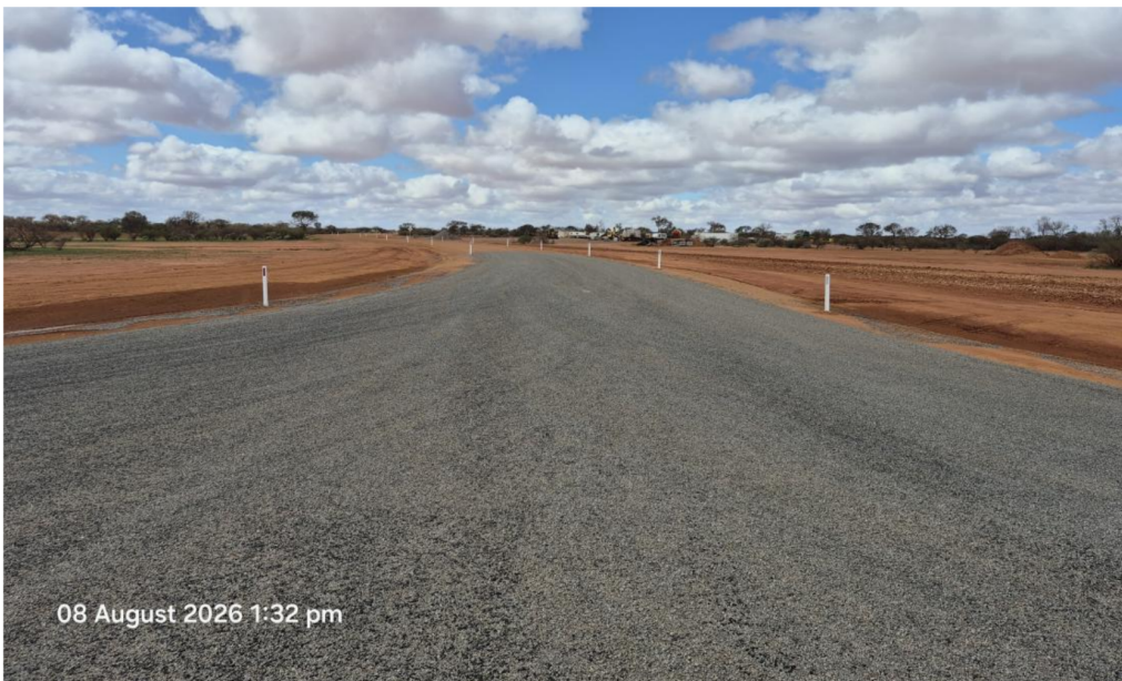
Work Area 4 - Landor Mt Clere Rd intersection
