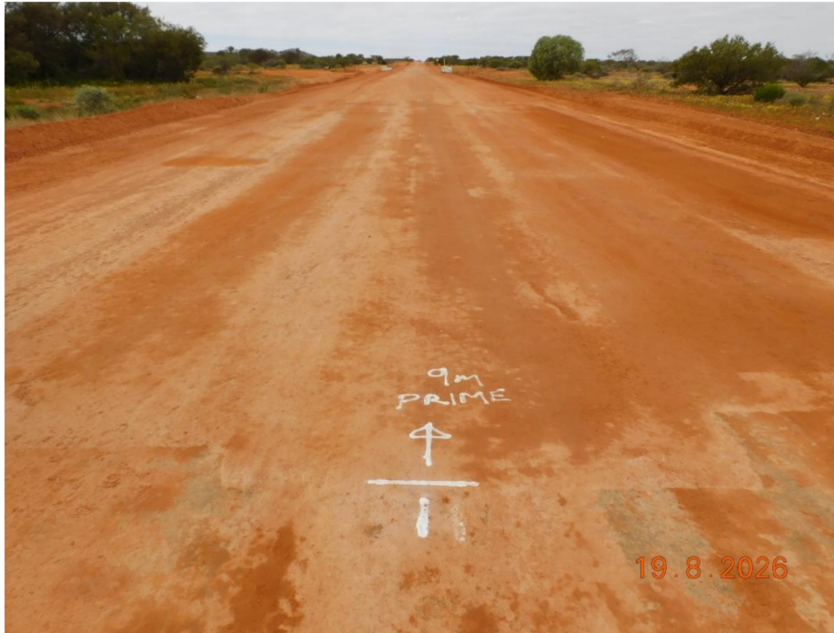
Cement stabilised floodway final trimmed
