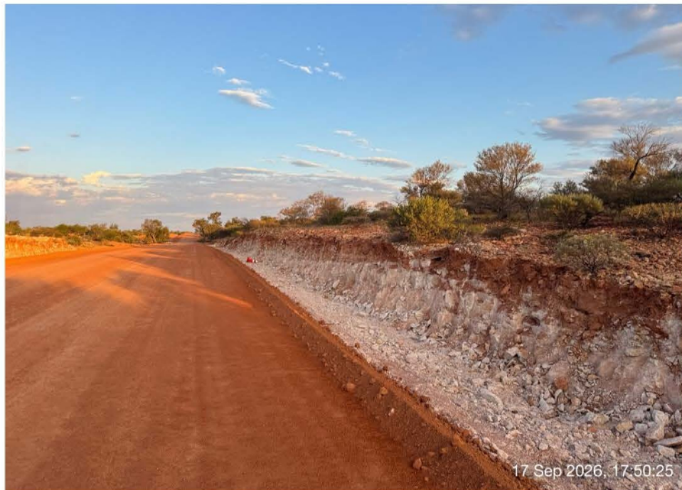
Rock removal to establish new drainage
