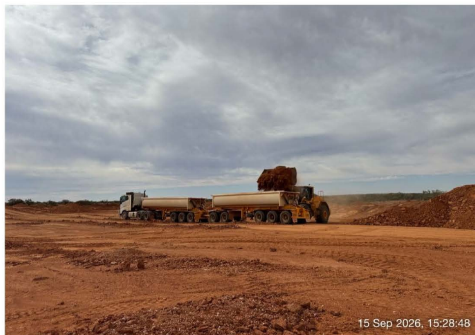
Basecourse material loading out
