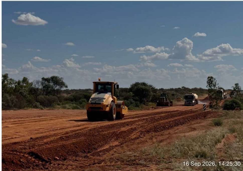
Basecourse mixing and compaction in progress
