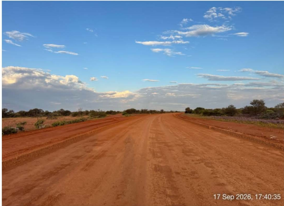
Basecourse ready for final trim
